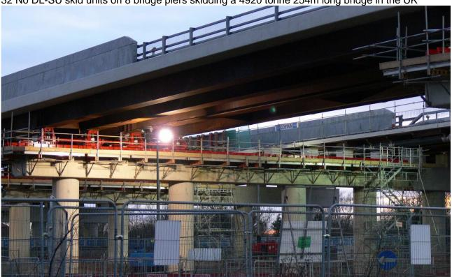
The main features of the DL-SU synchronous jacking and skidding systems are as follows:
